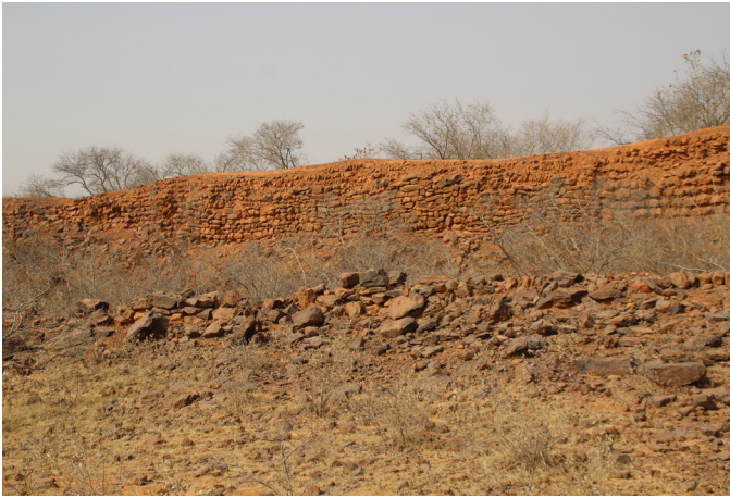
Figure 2: An outside view of Surame's wall from one of the most preserved sections. Author's photo 2019.
