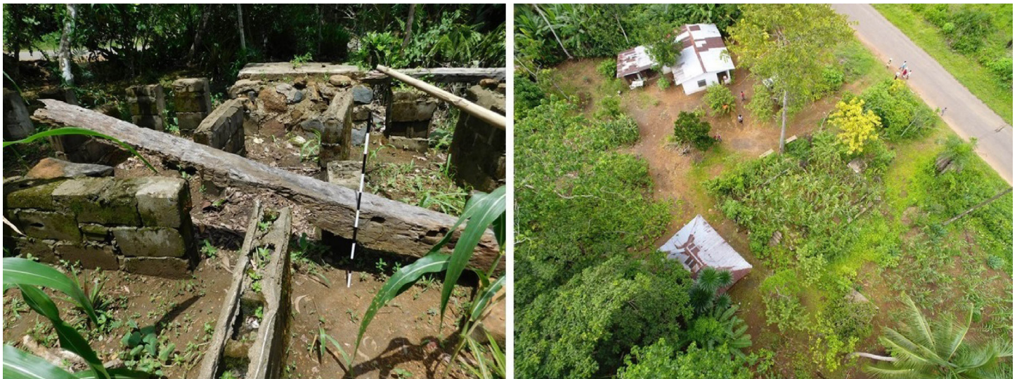
Figure 2: Remaining foundation columns and structural beams of the Padmore household (left). An aerial view of the Padmore property with the ruins of the former family house visible in the midst of a small plot of corn (right). This was likely the third house built by the Padmore family, and it underwent several refurbishments and upgrades before it was shelled and eventually destroyed in the twenty-first century. Photographs by Matthew Reilly.
