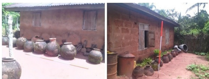
Figure 3: Ceramic pots arranged for collection of rain-water from the roof. (photo E.E. Okonkwo)
